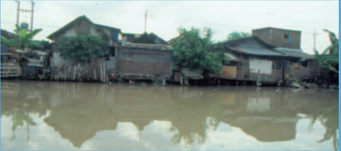
Many of the tightly packed houses that line the bank of the Brantas use the river as a rubbish dump and open sewer.
